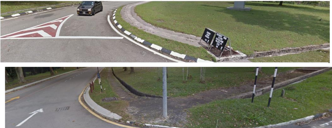
Figure 2: The picture above shows the pedestrian walkway provided ended at the drainage too. Not well connected and unsafe for pedestrian. (Source: Author, 2021).
