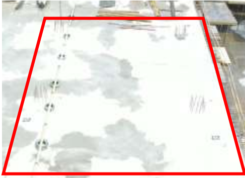
Figure 5b Concrete slab monitoring area
