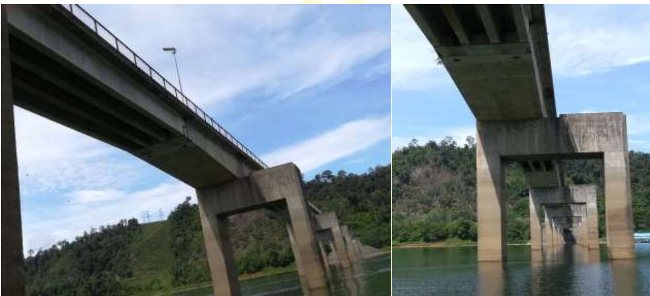
Figure 1: The structure of Sungai Perak Reservoir Bridge
