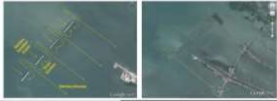
Figure 3. The failure in coastal protection engineering (Sugianto, 2019).
